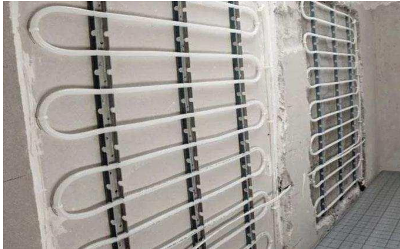
Figure 2 – Water wall heating system
