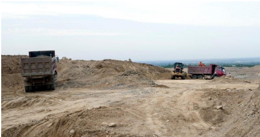
Figure 3 – Filling of depressions in the earth's surface
